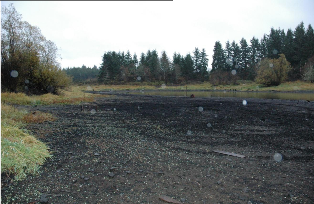
Fill pad edge at east end of Goose Lake, looking south
